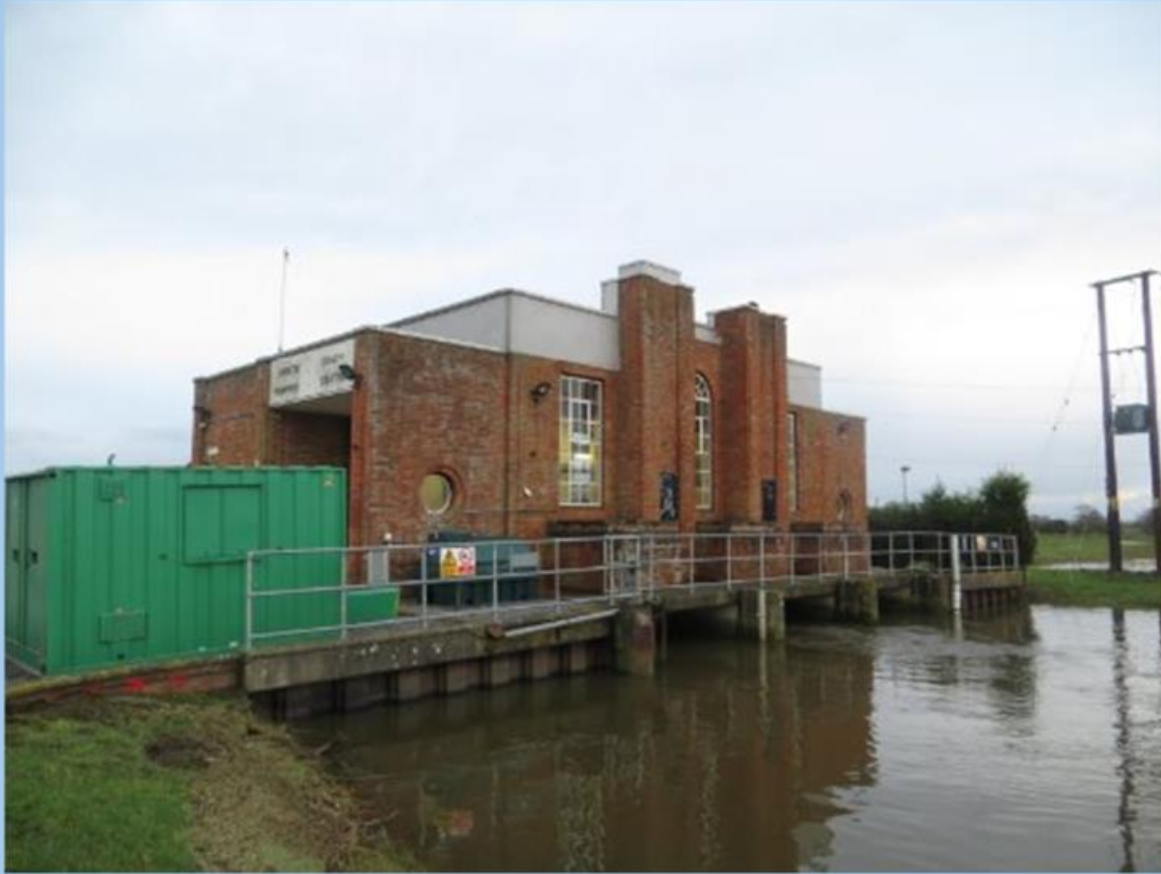
North Drain Pumping Station
