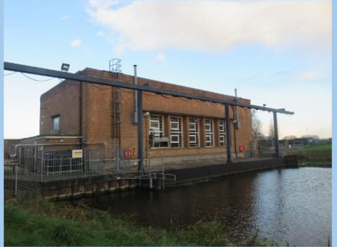
Gold Corner Pumping Station
