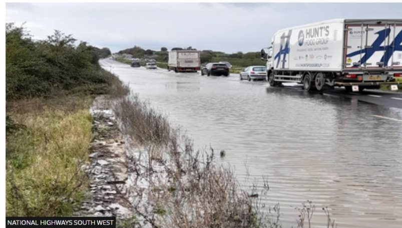
NATIONAL HIGHWAYS SOUTH WEST The A303 in Somerset has flooded after heavy rainfall
